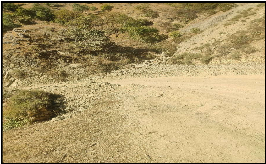
Existing Road Condition
